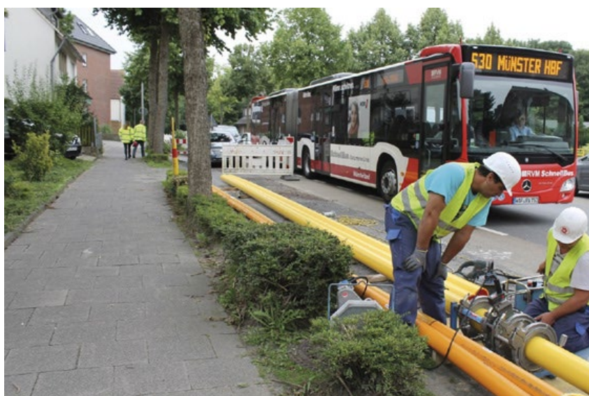
Figure 2. Installation of PE pipes [8]
