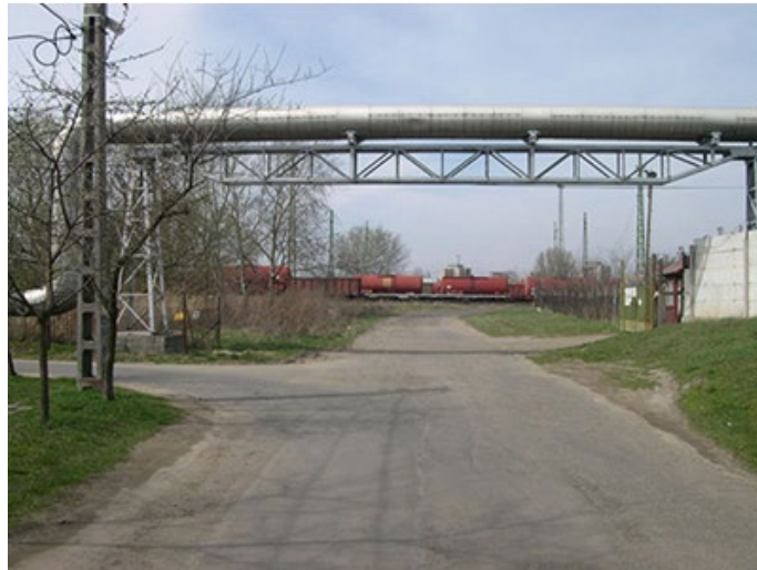
Figure 1. Welded support steel structure of district heating lines
