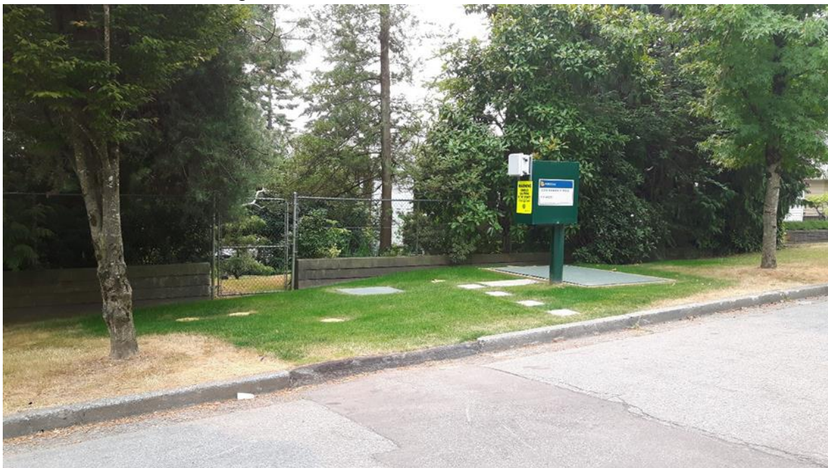
Figure 16. New Station Installed
